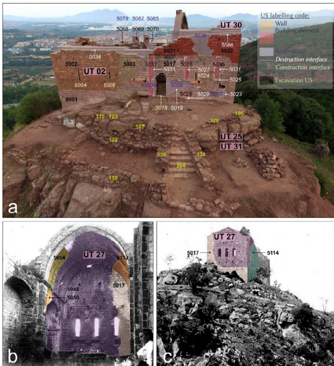
Fig. 2. Aerial view of Sant Genís de Rocafort after fieldwork carried out in 2020 (a), and photographic vestiges from the beginning of the 20th Century (b-c) [35]–[36]. Interpreted relations between US and UT are recorded in Table III.
